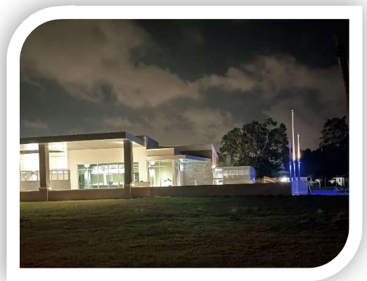
The City of Palmetto began construction of 20,000 gross square foot Palmetto Police Department in Spring 2022 and will open in the early Summer of 2023.
